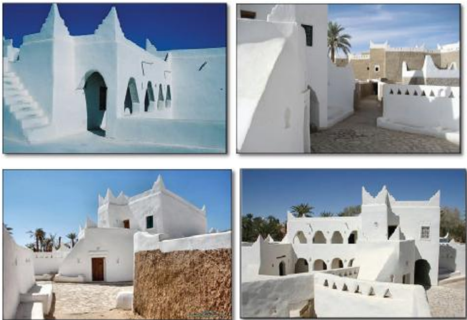
Figure 1 : Some examples of houses in the old city of Ghadames
